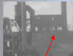
ESP in Operation Prior to Precip Filter
