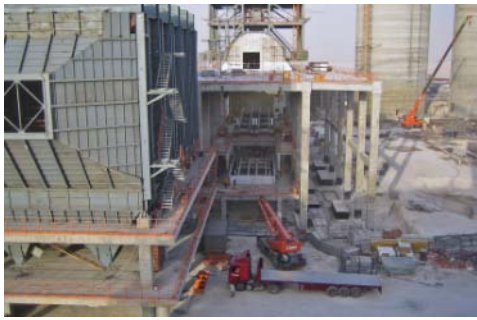
View along the ESP onto the 2-stage mobile structure at Hofuf #5
