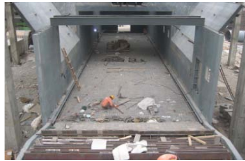
Covering the air beams with gate plates
