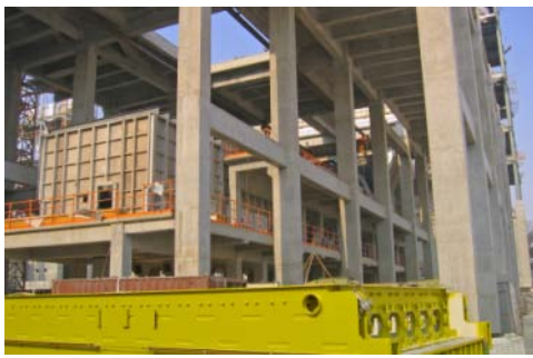
Preparations of crusher installation
