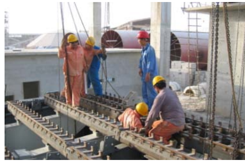
Installing the air beams on a width of 6.8 m
