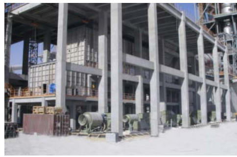
Cooling fans in position – shortly before start-up
