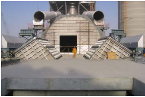
Burner platform with twin TA-offtakes and kiln hood in background
