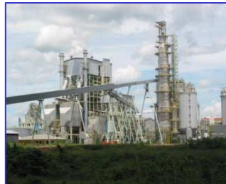
Digester- ODL plant
